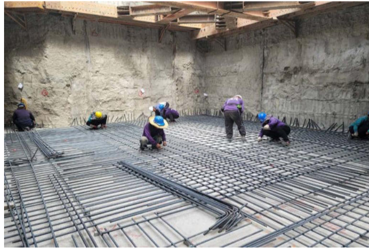
筏基鋼筋綁紮
